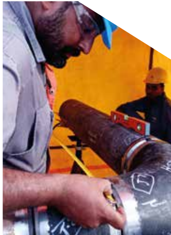
Fabrication & Erection (Steel Structure & Piping)
